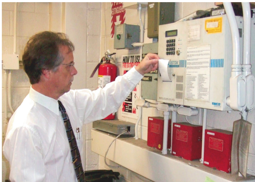
Jeffrey Tews checks water-level readout from the central repair garage underground tank monitoring system. The system's more-accurate readouts have replaced the "sticking the tank" checking method.
